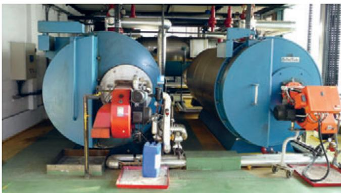
The old heavy oil boiler to be replaced
